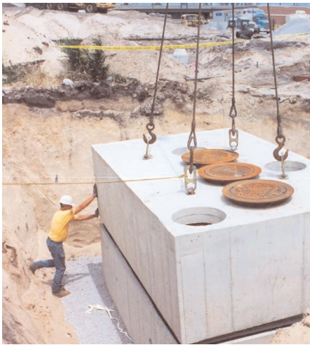
Award-winning Virginia Street Storm Sewer installation
